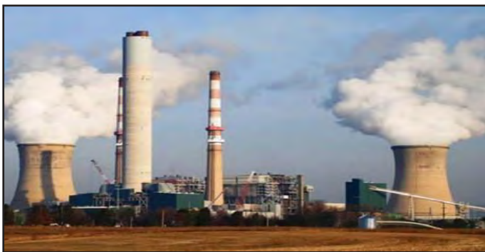
Fig. 1: Shows a Photograph of Self-Supporting Steel Chimneys Located in an Industrial Plant
