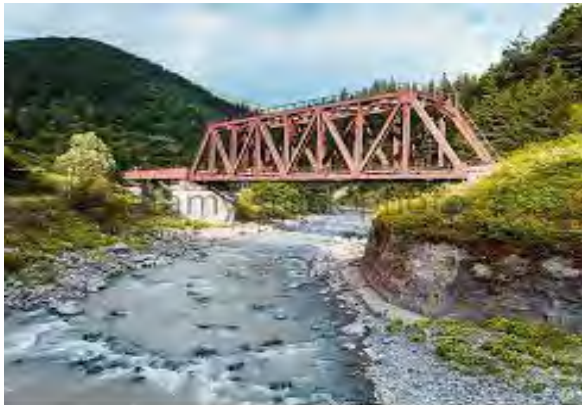
Figure 1. Structure of Iron Trestle
