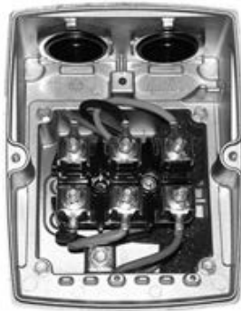
Figure 5.9 Terminal box of an asynchronous motor
